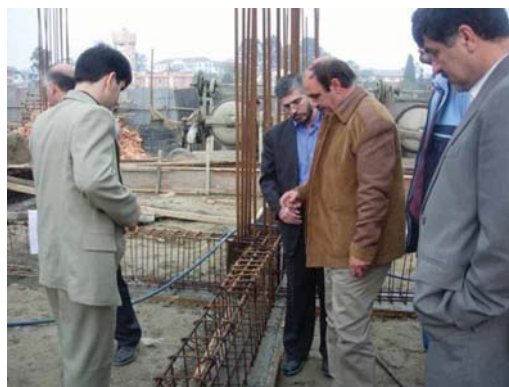
Visit at building construction site
